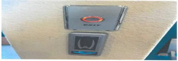
**Clubhouse Exit** A new exit button was installed at the front door of the Clubhouse which allows people to exit without using an Access Card. This exit button is active 24 hours a day. The Access Card scanner is remains active as well.
